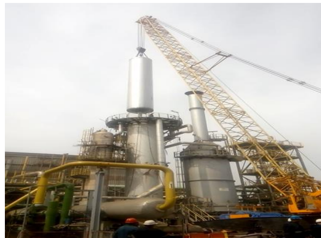
Figure 1. Ammonia Converter Basket Revamp
