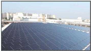
In order to build business model, which contributes in national power saving movement, LG Ltd. has developed LG photovol taic power generation, which sizes about 43,410 m² with capability of 2,988kWp. Since July 2012 when the installation finished, it creates 12.9GWh accumulatively. (by 2015 Dec)
