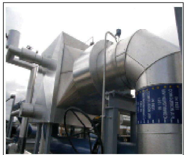
Figure 7: Combustion Air Pre-heater on Incinerator
