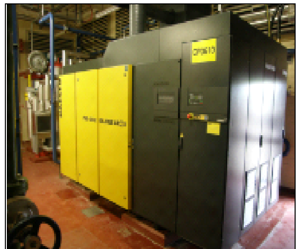
Figure 6: Site Air Compressor with Heat Recovery
